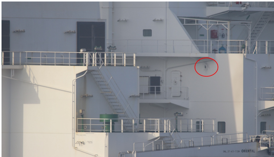
Damage from Iranian fire on the RICHMOND VOYAGER (Source: USCENTCOM)
