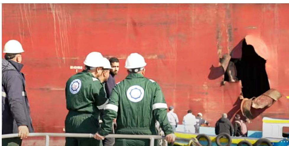
Damage on the bulk carrier ZOGRAFIA which was struck by a missile in the southern Red Sea on 16 January (Photo: Social media)
