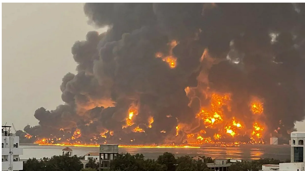
Oil storage tanks on fire in Hudaydah following an Israeli strike (Photo: Almasirah Television)
